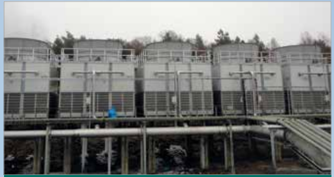
Plant after the replacement with MITA modules
