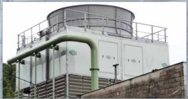
Plant after the replacement with MITA modules
