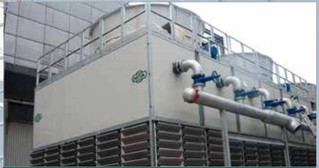
Plant after the replacement with MITA modules
