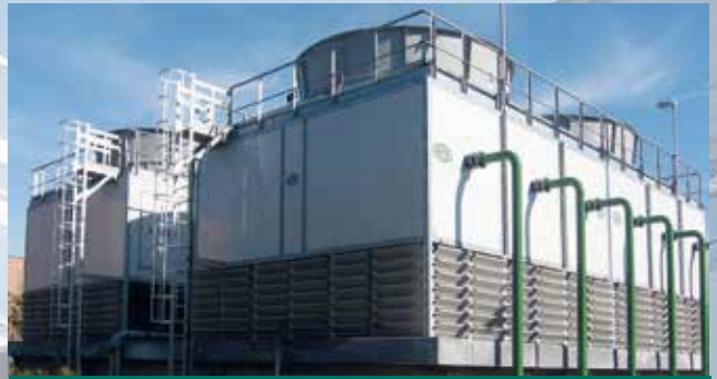
Plant after the replacement with MITA modules
